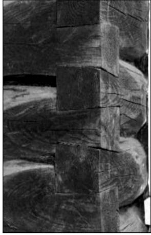
Rounded wall logs squared and dovetailed corners.
